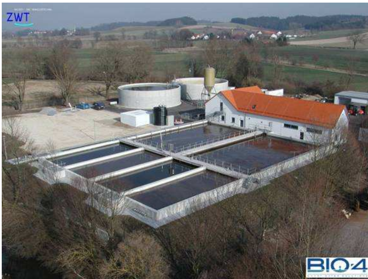
BIOCOS®- 10.000PE plant of the community Petershausen in Germany
