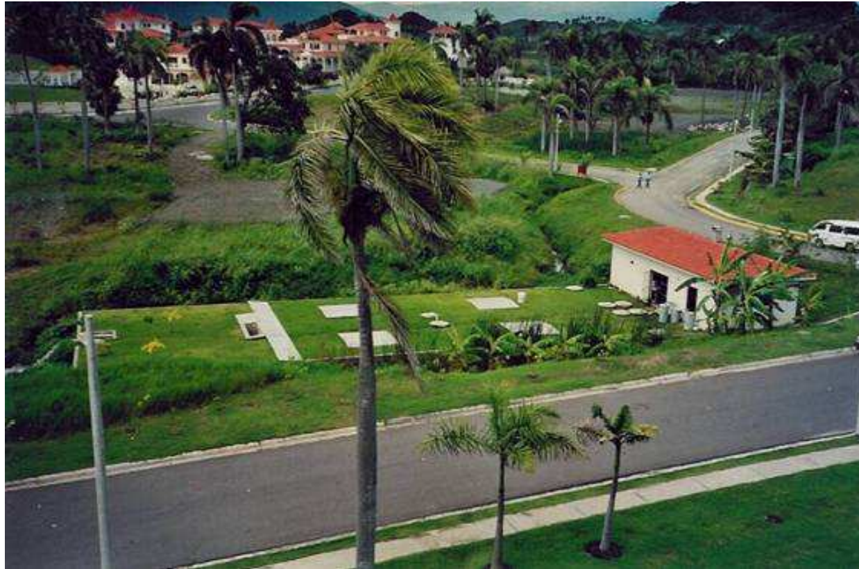
Resort Cofresi Beach Consortium, Puerto Plata Dominican Republic. Covered construction 4.000 PE
