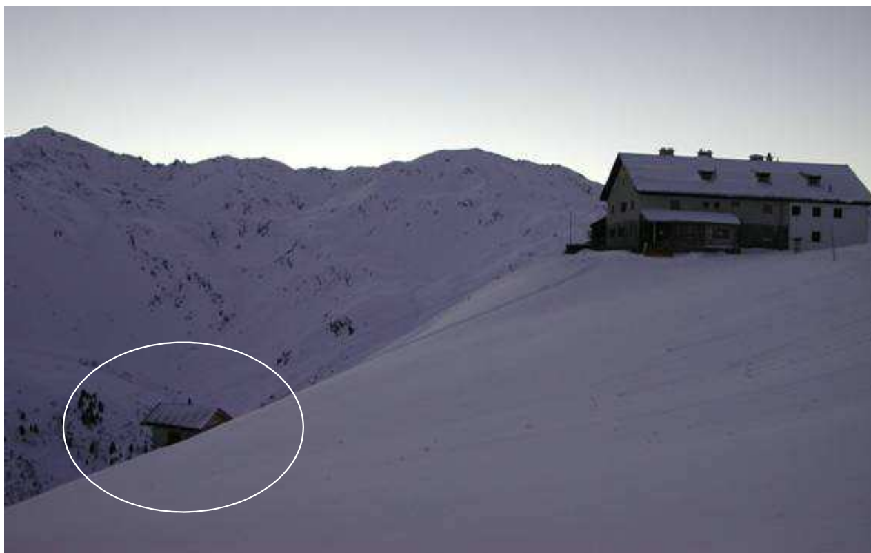
BIOCOS plant for 100PE in an alpine refuge 365 days operation – sewage temperature of about 5°C
