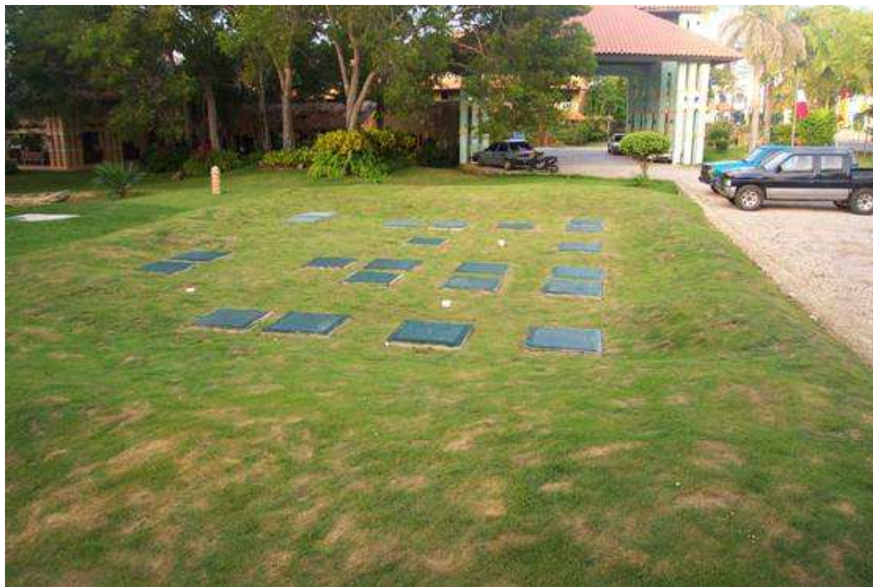
Hotel Estrella Azzura, Cabarete, Dominican Republic. Covered construction 750 PE
